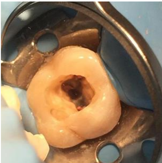
Fig 5: Access to the chamber showing an evident perforation in the pulpal floor.
